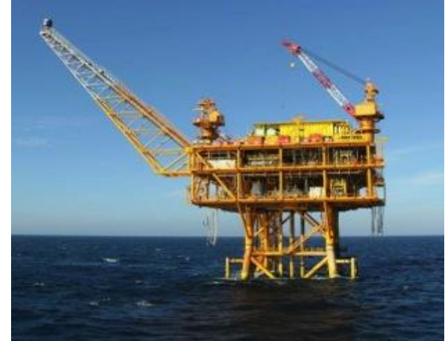
Topside lifted June 2013, installation completed June 2013
