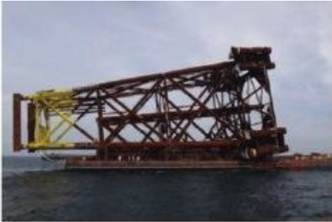
Jacket Installation July 2012
